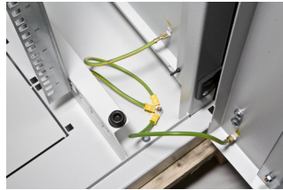
internal earthing of all cabinet parts
